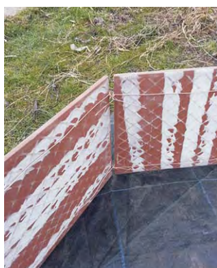
Step 6: Join by twisting wire ends, edge to edge.
